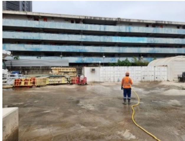
Photo 8 – Watering on the main haul road
